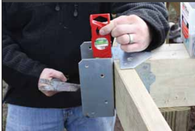
Position & Plumb Splash Handrail Bracket
