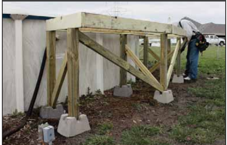
Typical 2"x4" Diagonal Bracing Board Layout
