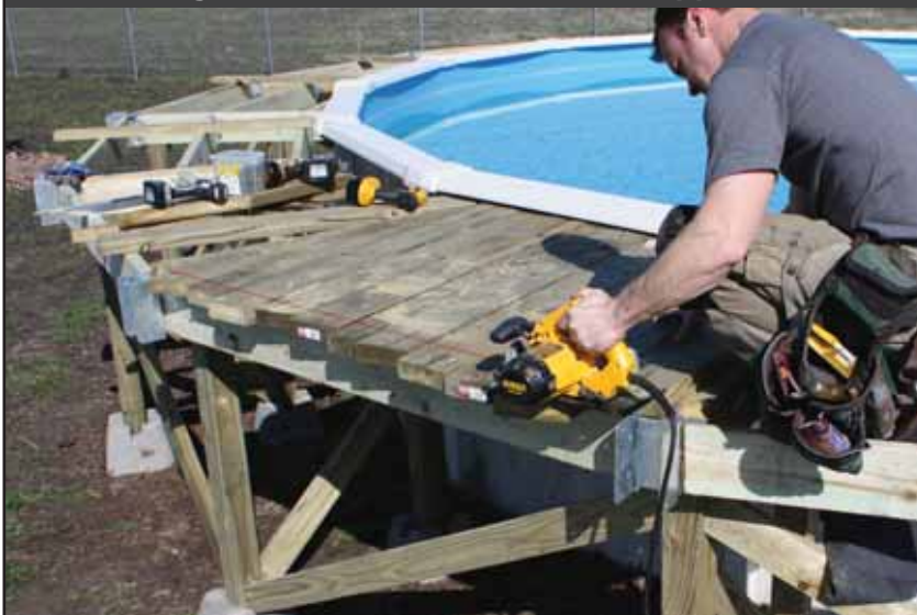
Trimming Surface Boards Flush with Support Frame
