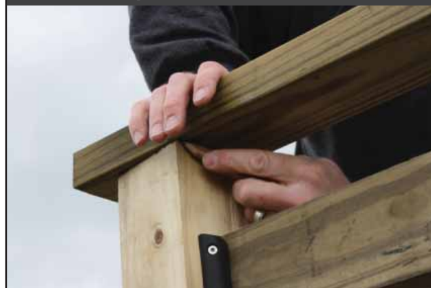
Mark Top Handrail Board for Cuts
