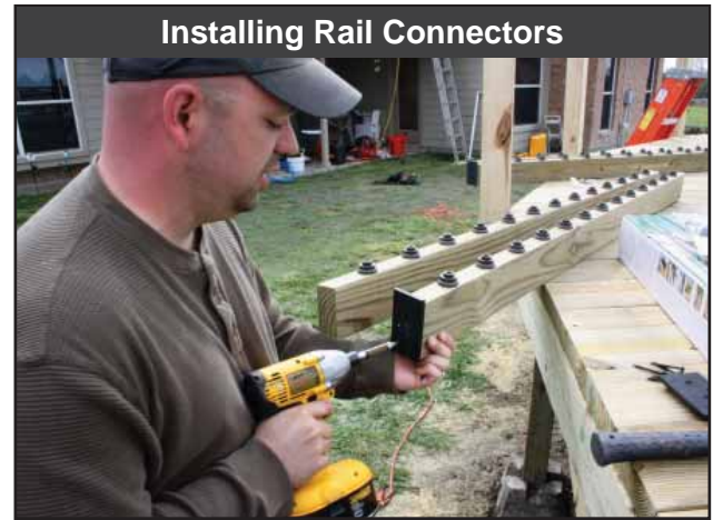
Positioning Bottom Rail Board
