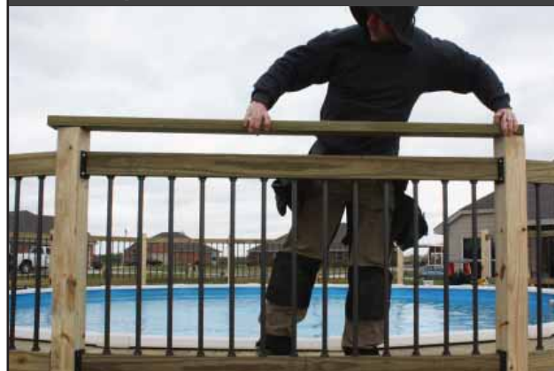
Place Top Handrail Board over 4"x4" Posts
