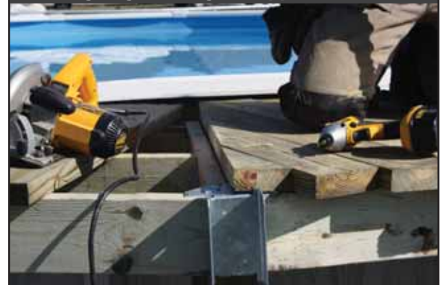
Aligning Decking to Support Boards
