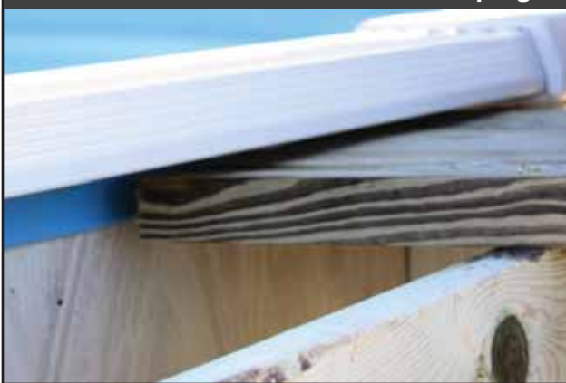
Surface Board Under the Pools Coping
