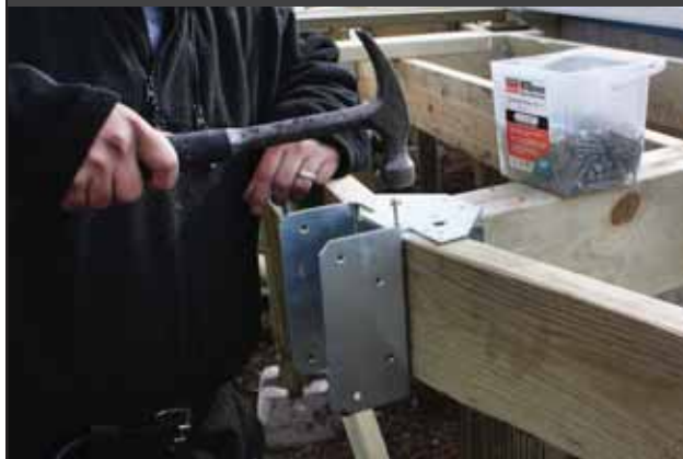
Securing Splash Handrail Bracket
