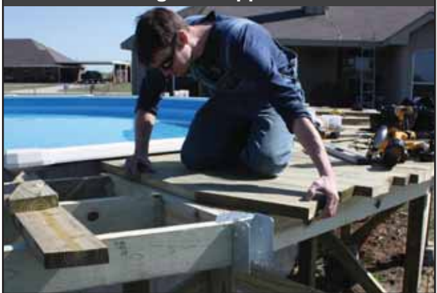
Aligning Surface Boards with Edge of Support Frame
