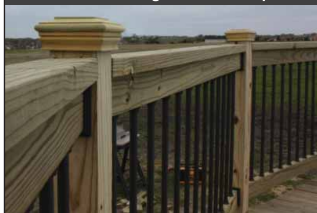
Finished Railings with Post Caps
